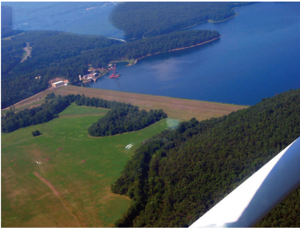
Figure 30. CAW Property Near the Intake Structure
