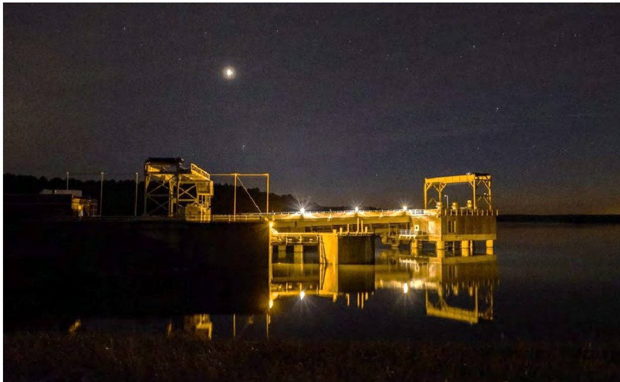
A planet shines bright above the Lake Maumelle intake.
