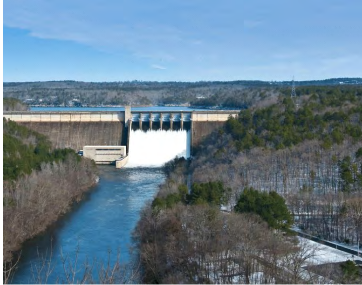
Dam at Greers Ferry
