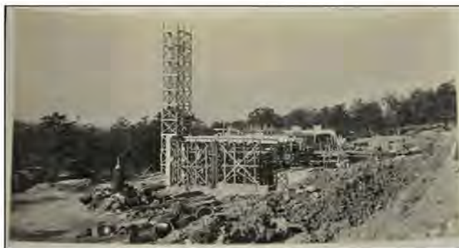
Oct. 29, 1937 – Ozark Point Plant under construction.
