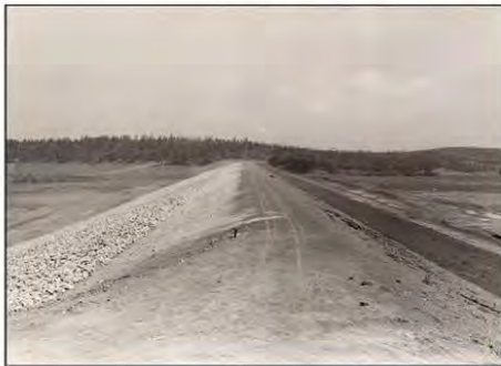
1957 – Lake Maumelle construction.
