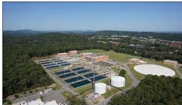
2017 aerial photo of the Wilson Plant.
